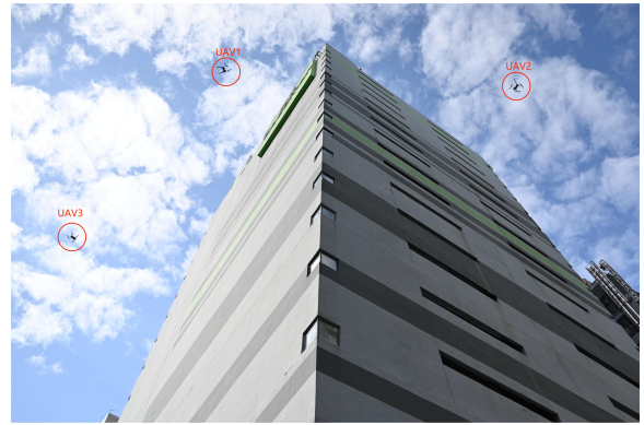
Fig. 3. Three UAVs cooperative inspection for a logistics center building.
