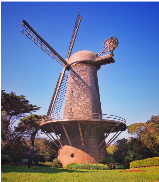
Fig. 1. Windmill with fantail-driven feedback
